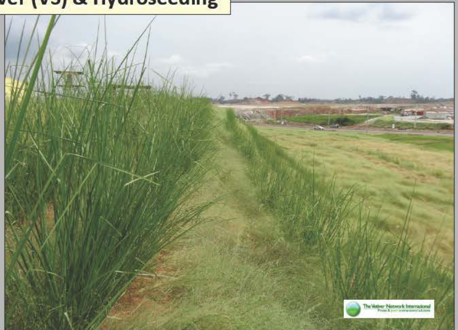
Established Side Slopes using Vetiver (VS) & Hydroseeding
