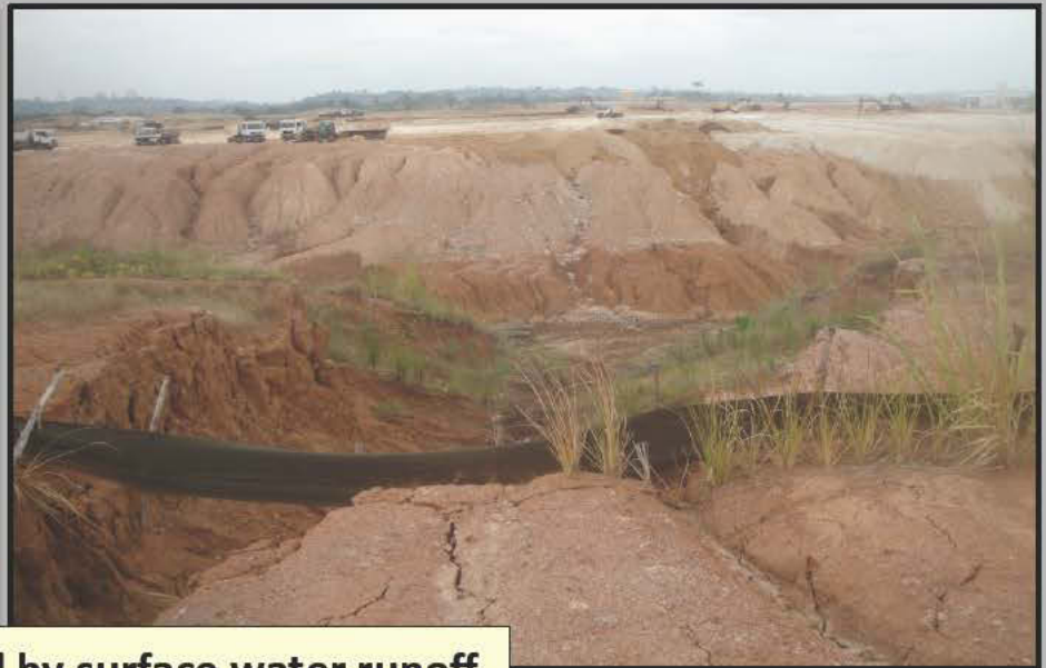
Excessive Erosion caused by surface water runoff
