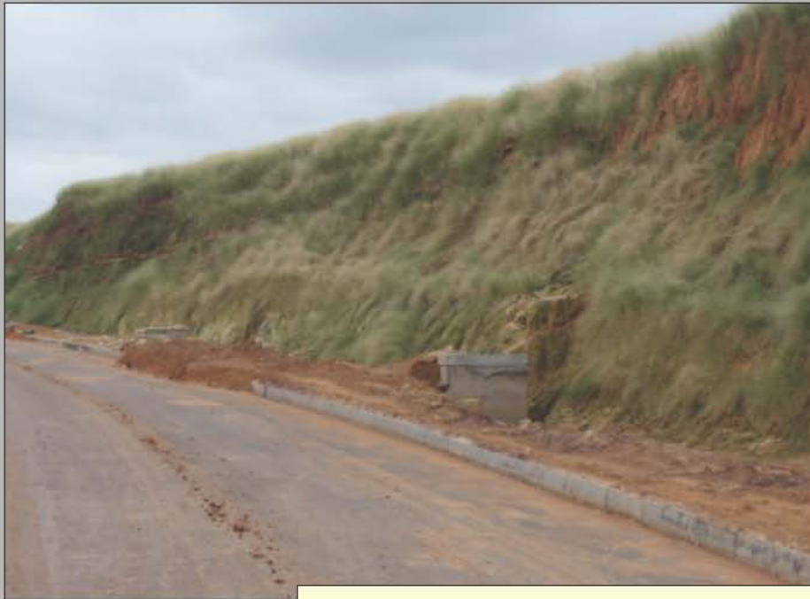
Established Side Slopes using Vetiver (VS) & Hydroseeding
