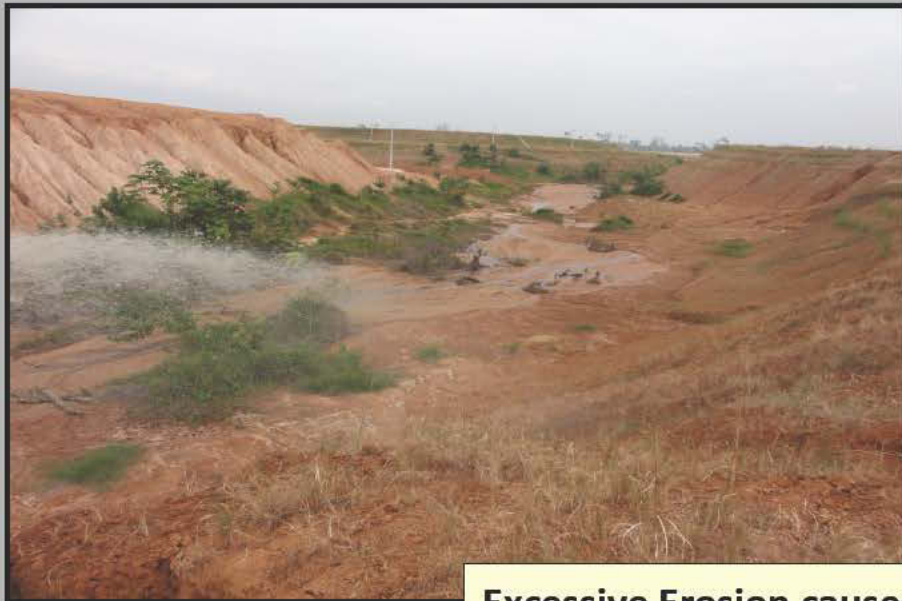
Excessive Erosion caused by surface water runoff
