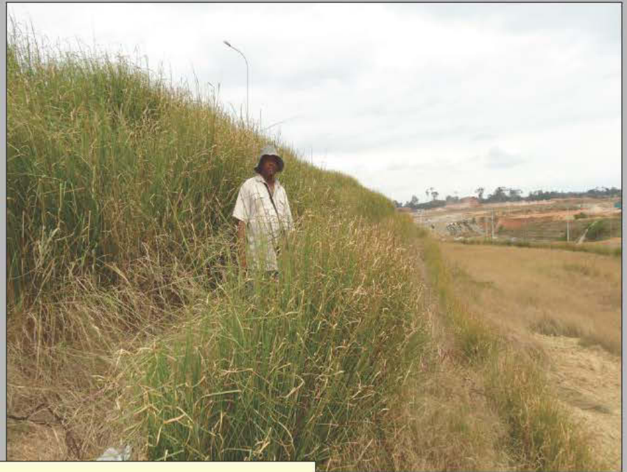
Established Side Slopes using Vetiver (VS) & Hydroseeding
