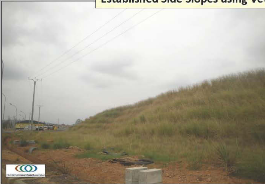
Established Side Slopes using Vetiver (VS) & Hydroseeding
